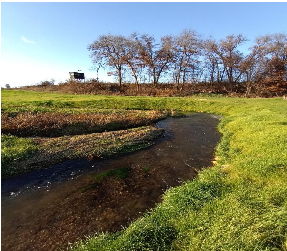
A field road existed between the tree line and stream so bank tapering was limited, but enough rip-rap was utilized to assure bank stability. A backwater area that was created is visible in lower picture.
