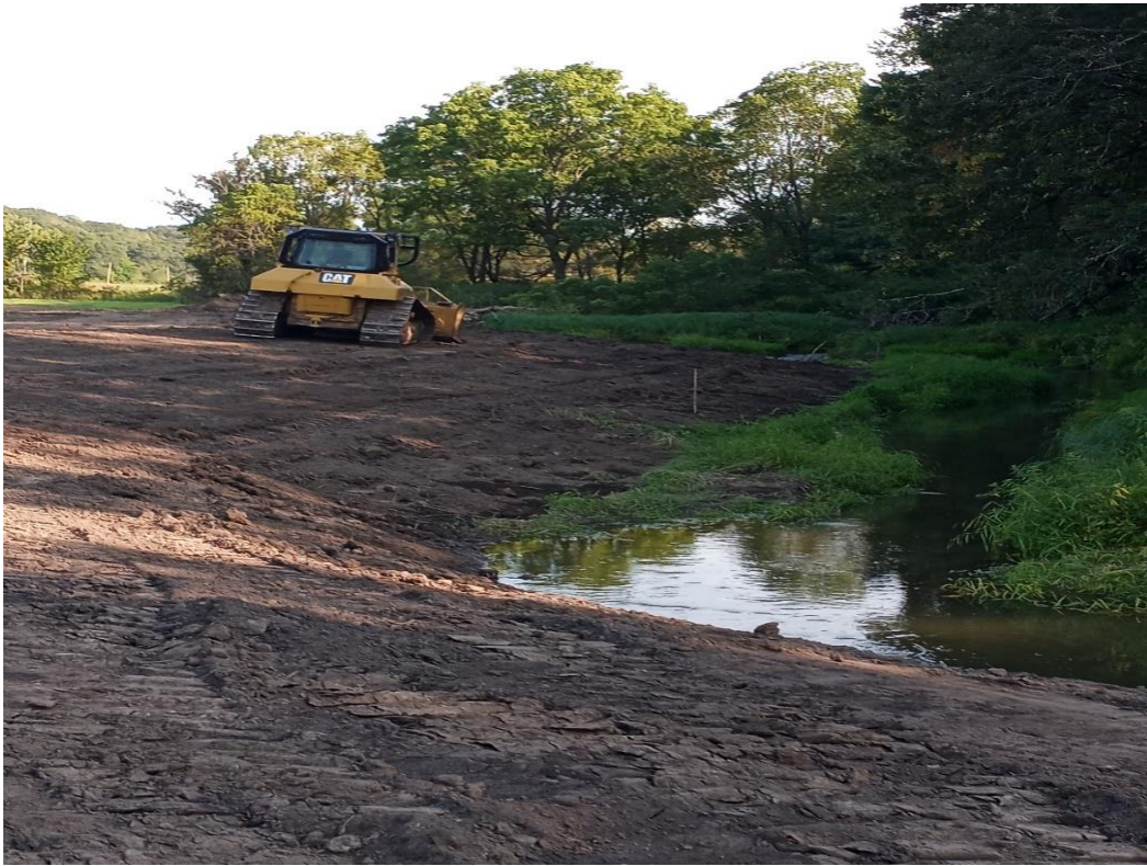
The previous photos show a bank being tapered and rip-rap being installed. The above photo shows the final shaping being done. The lower photo shows a weir that was installed with several log deflector sets that were installed above it.
