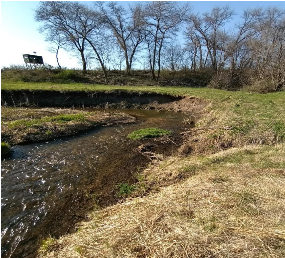
A field road existed between the tree line and stream so bank tapering was limited, but enough rip-rap was utilized to assure bank stability. A backwater area that was created is visible in lower picture.
